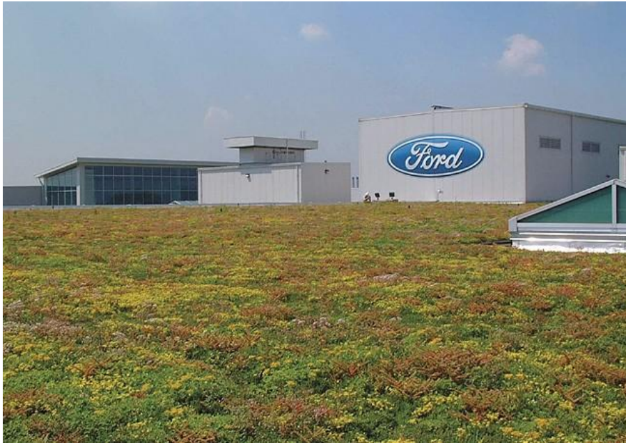
Above: The Ford Assembly Plant in Michigan, US
